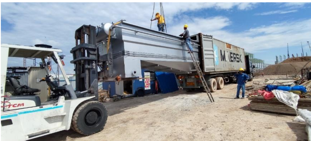
Figure 2: Unloading process of DAF2-050 from container
